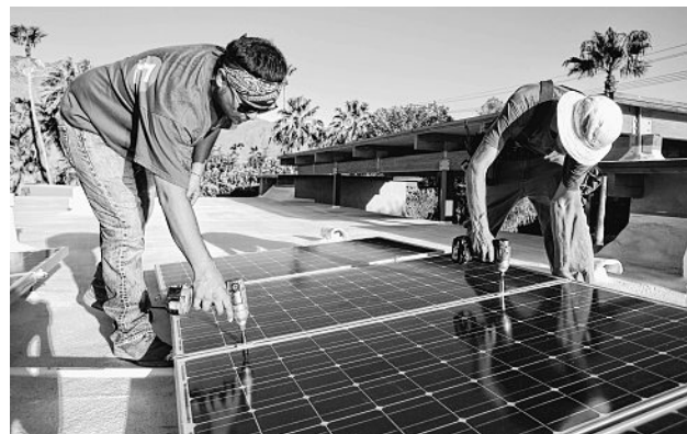
A Hot Purple Energy crew install solar panels. CRYSTAL CHATHAM/THE DESERT SUN
